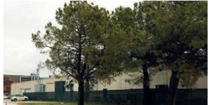
UFLEX - Factory in Tregnago
