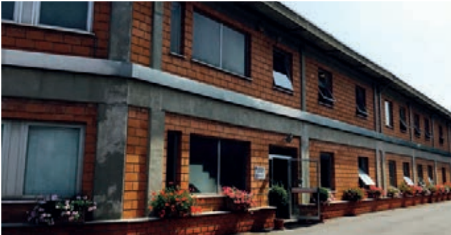
UFLEX & ULTRAFLEX - Headquarter in Busalla
